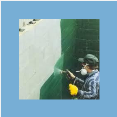
Polymer Waterproofing Service
