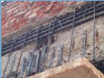
Retrofitting Restoration Service
