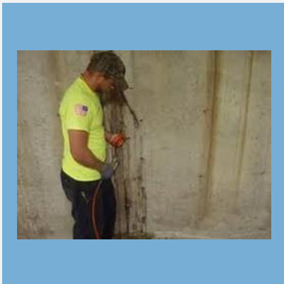
Structural Crack Repairing Services
