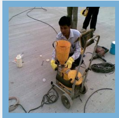
Injection Waterproofing Service
