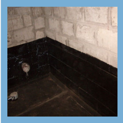
Bituminous Waterproofing Service
