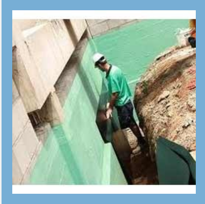
Wall Waterproofing Service
