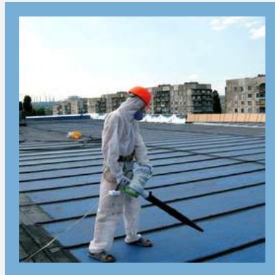
Waterproofing Treatment Service
