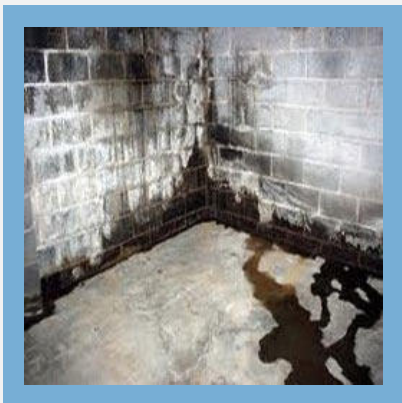
Basement Waterproofing Service
