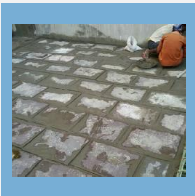
Box Type Waterproofing Service
