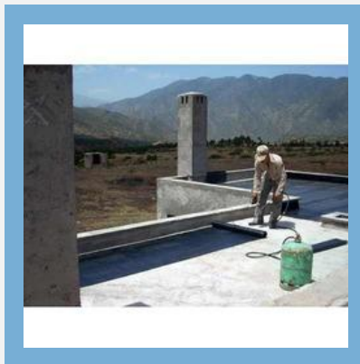
Terrace Waterproofing Service
