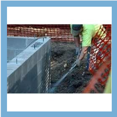
Foundation Wall Waterproofing Service
