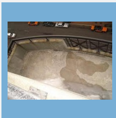
Balcony Waterproofing Service
