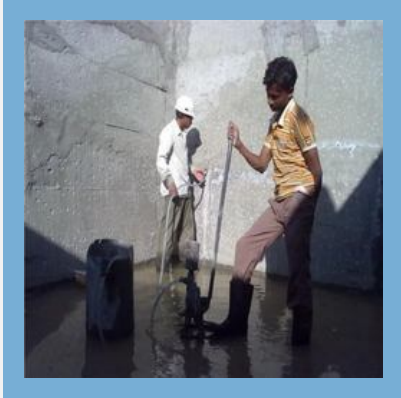
Water Proof Grouting
