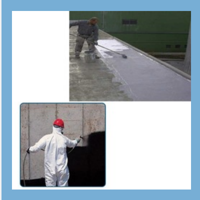
Bituminous Emulsion for Retaining Wall
